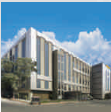
Switchgear Factory, Mumbai
