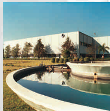
Switchgear Factory, Ahmednagar
